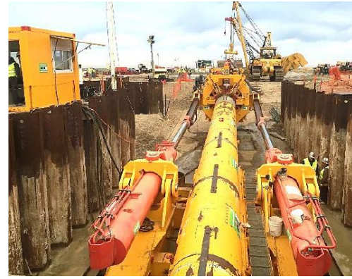
Plate 3.4: Direct pipe thruster equipment at the landfall compound
